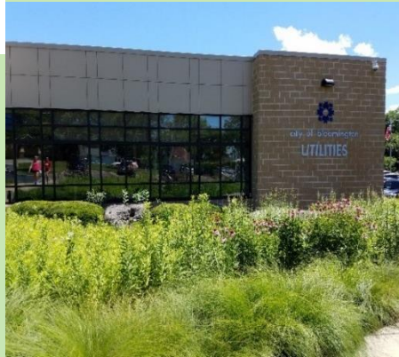
Figure 7.3 Rain Gardens can be designed to blend with a building’s landscaping.
