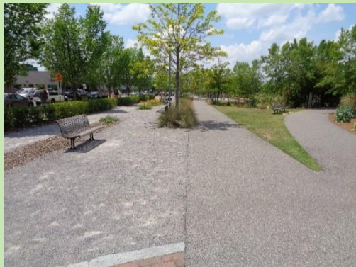
Figure 7.6 Permeable Pavement incorporated into sidewalk design
