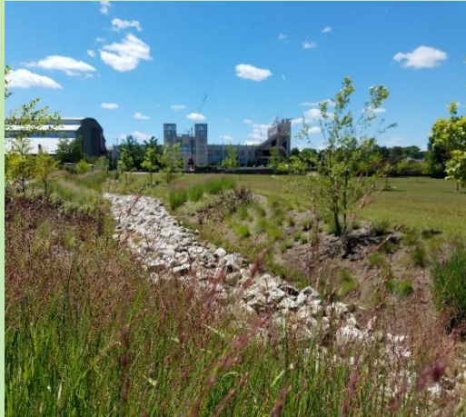
Figure 7.4 Example of Dry Water Quality Swale
