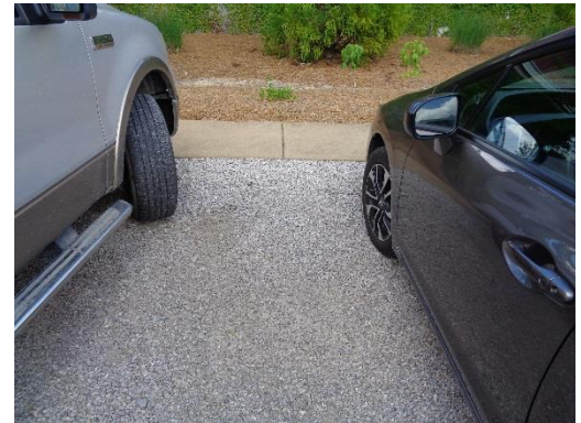
Figure 7.4 Permeable Pavement installed in a parking lot application
