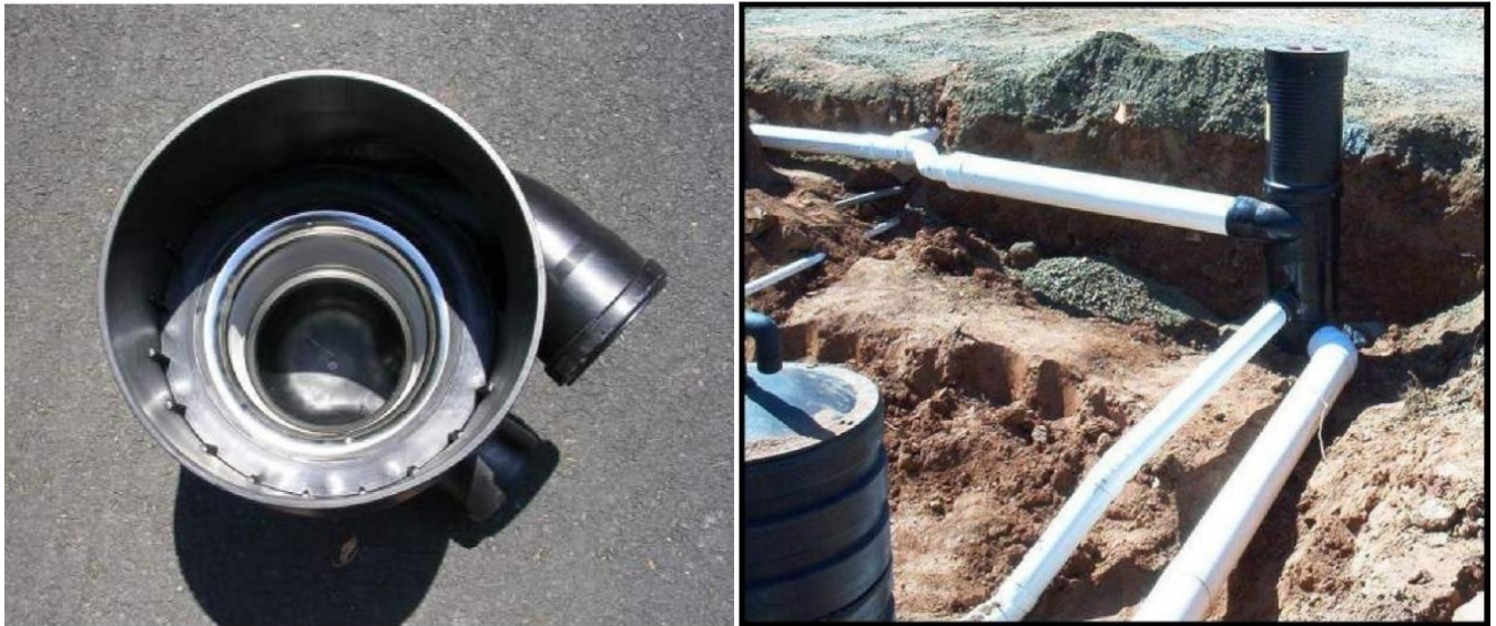
Figure 7.15 Interior of Vortex (left) and Installation of Vortex Filter Prior to Backfill (right)
